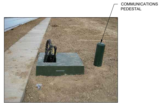
GROUND SLEEVE SIDE VIEW
